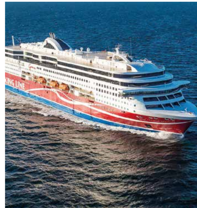
The EMMA energy management system used on board the Viking Grace reduces the ship's fuel costs and emissions by about 5 percent.
