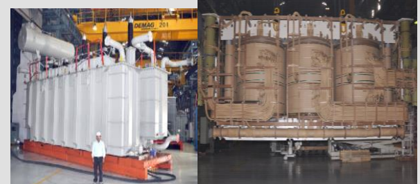
570 MVA Generator Trafo for Bangladesh thru ABB Singapore
