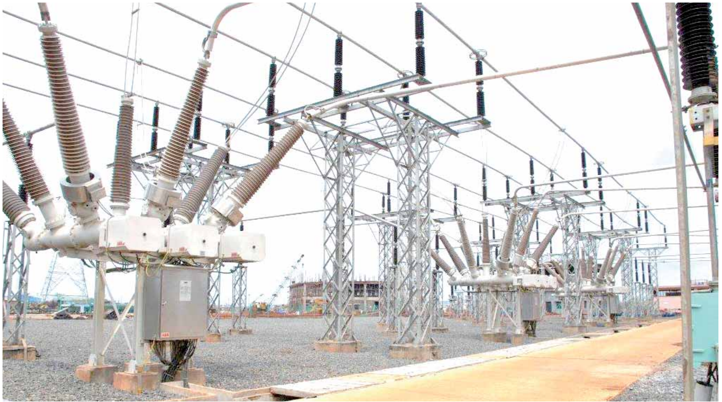
PASS module at GMR Energy's switchyard
