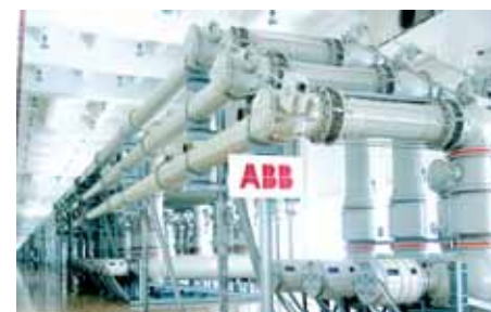
220 kV gas insulated substation
