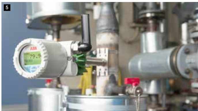
Figure 5: TSP341-W noninvasive temperature measurement
