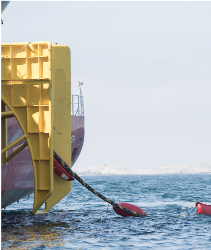
The new DC power cables to the Troll A platform, lowered into water just outside Kollsnes.
