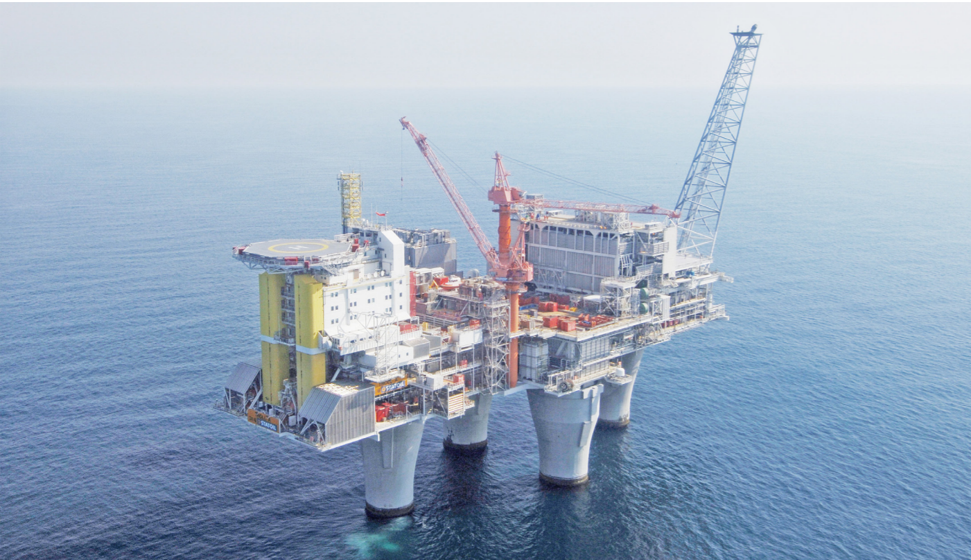
For the Troll A platform, Statoil has twice selected power from shore with ABBs direct current system, HVDC Light, to run gas compressors on board. Electrification is eco-friendly and cost-effective, and hence represents a shortcut to a more sustainable and profitable oil and gas industry.
