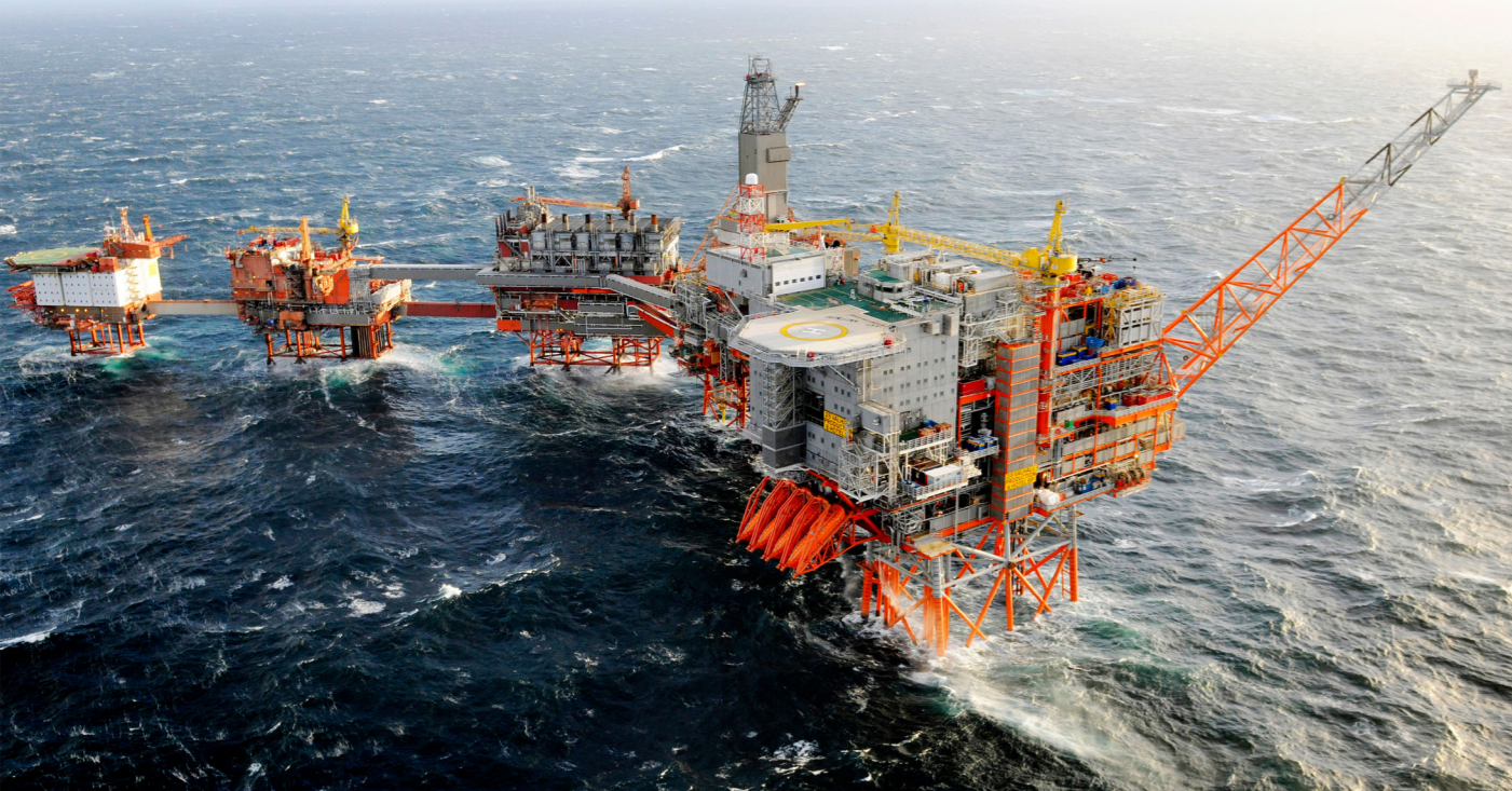
BP’s Valhall complex receives power from shore through a 292 kilometer long HVDC Light system from ABB.
