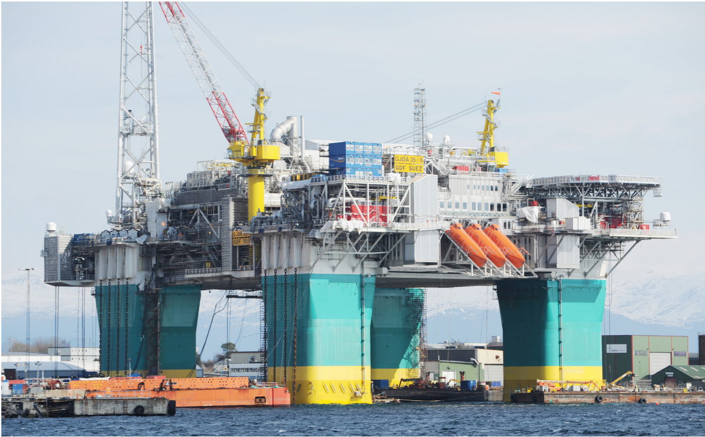
The Gjøa platform receives power from shore through a 100 kilometer long AC connection to Mongstad in Hordaland. This is from the preparation at Stord.
