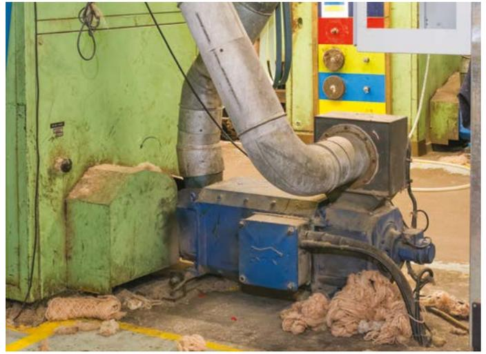
Old DC motors, prior to removal, shows the forced ventilation fan fitted as part of the closed ducted cooling system.
