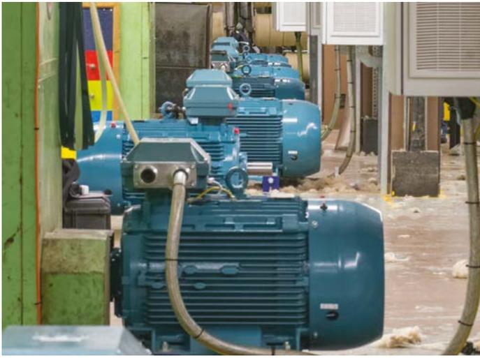
IE3 ABB motors, each rated at 75 kW, have replaced obsolete DC motors and eliminated costly cooling systems required by the DC motors.
