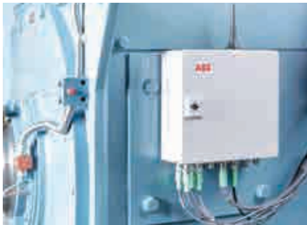
MACHsense-R is a remote condition monitoring solution for motors and generators.
