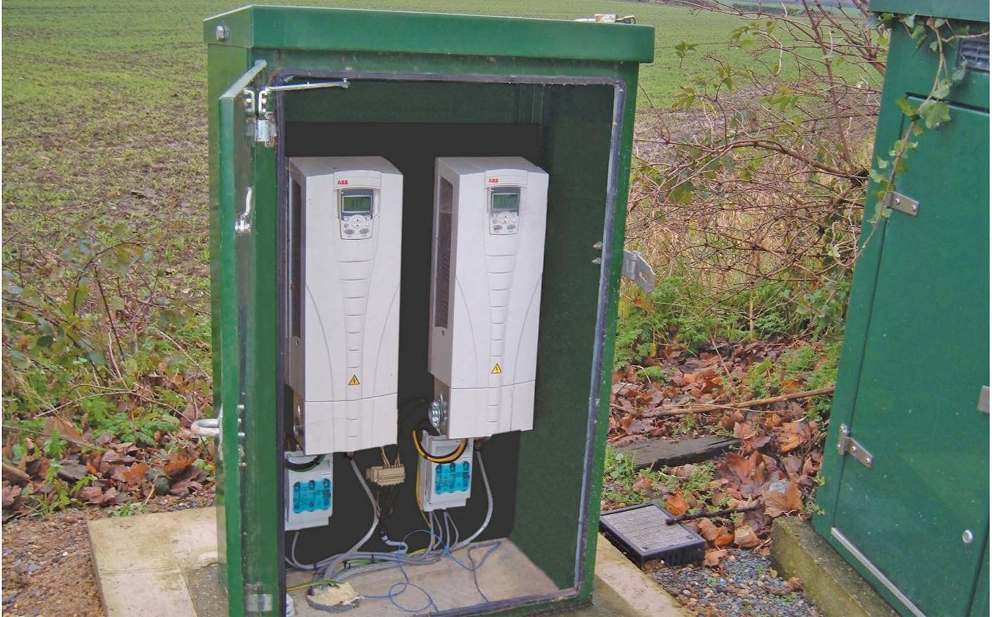
ABB standard drive range of low voltage AC drives used to create a synthetic three-phase supply
