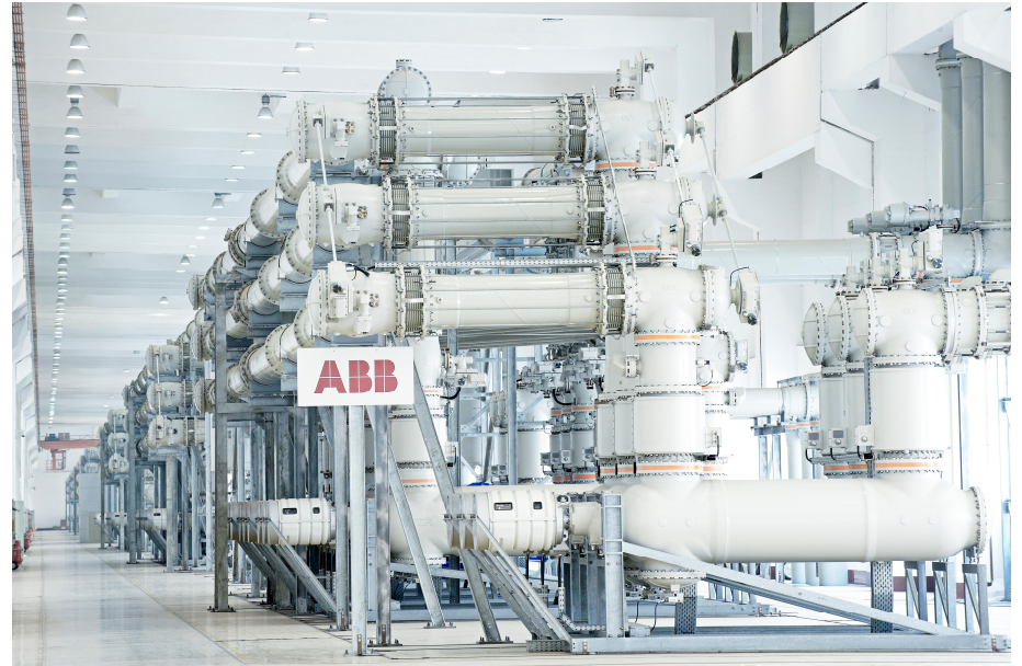
Large Gas Insulated Substation (GIS)
