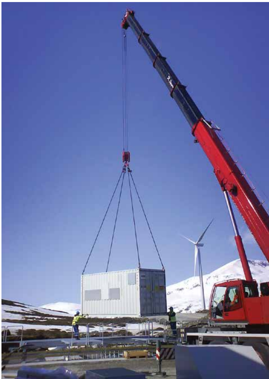
A crane positioning one of the PCS100 STATCOM containers into place
