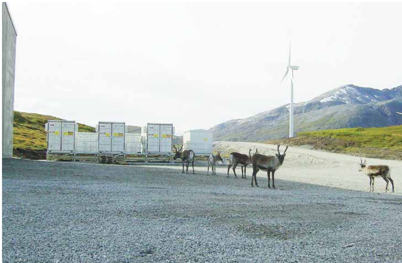
Three 2 MVar PCS100 STATCOM containers for a 54-megawatt onshore wind farm located in Fakken, in the far north of Norway
