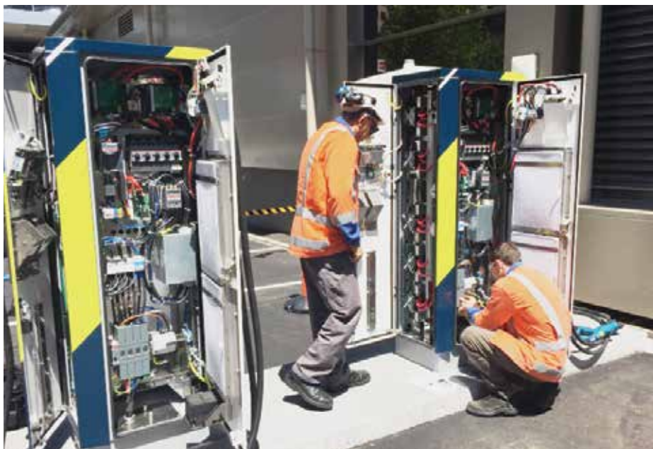
ABB’s engineers commissioning the chargers prior to launch
