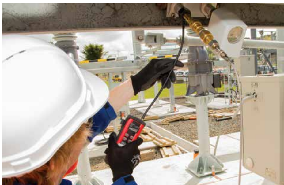
ABB service testing to ensure there are no leaks while filling the DCB.
