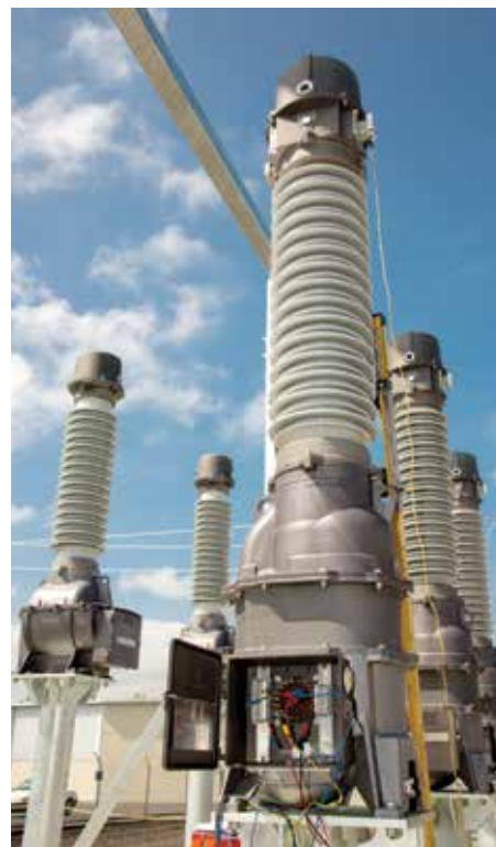
Installation and testing of current transformers.
