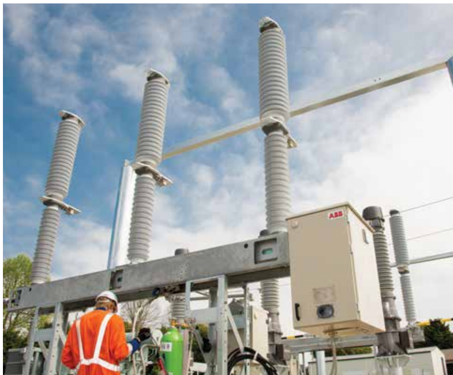
SF6 gas filling of the installed disconnecting circuit breakers (DCB).
