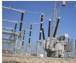
Shunt reactor
