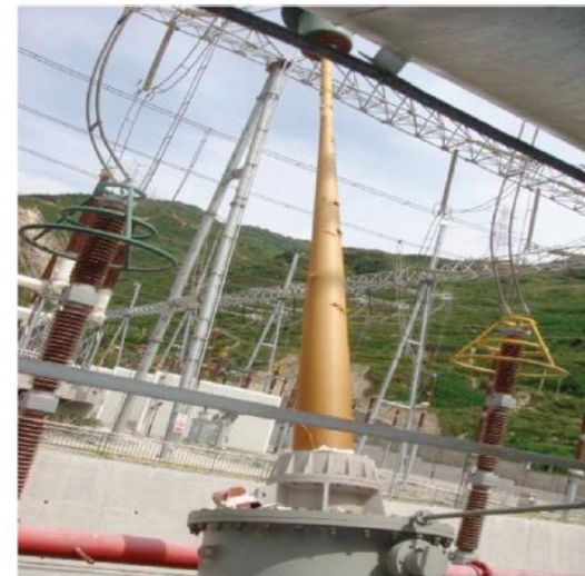
Figure 6. Bushing. 500 kV Transformer
