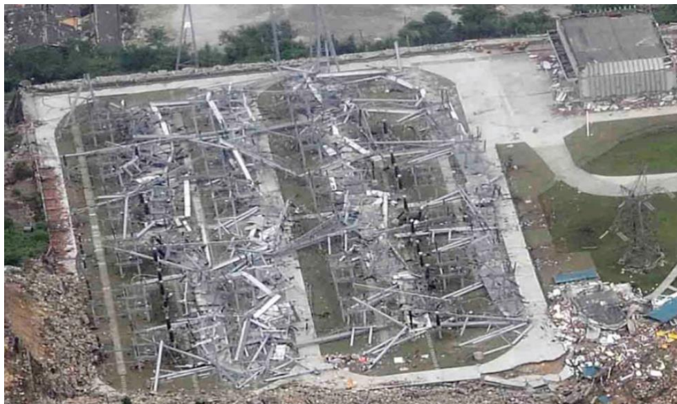
Figure 9. Destruction to Ertai Shan Substation, 220 kV, Yingzhou
