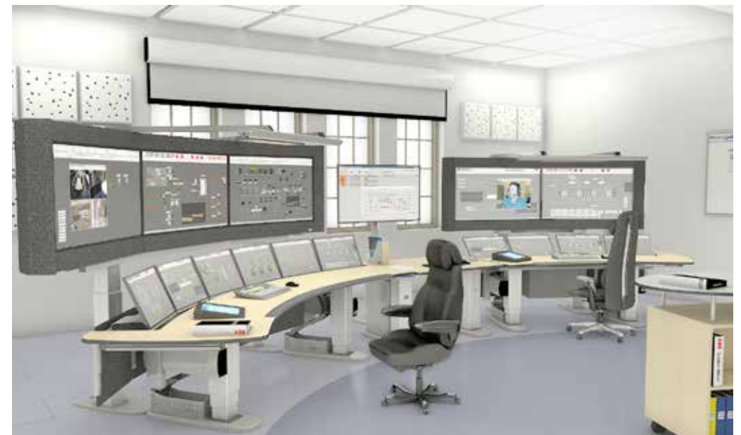
The control room at the Statoil-Hydro Tjeldbergodden methanol plant in Nordmøre, Norway. Warm spillwater from the plant is fed directly to a nearby fish farm. Wind measurements and temperature readings of the spillwater are integrated into the system.
