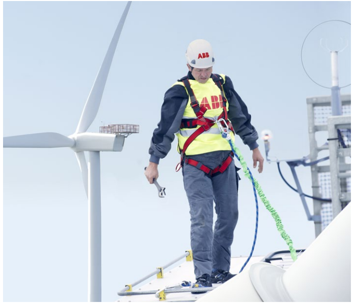
ABB field service engineer during commissioning
