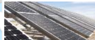
Established Shenzhen Power-One Renewable Energy; focuses on photovoltaic inverters and electric vehicle charging technology
