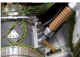
2008 Generator circuit breaker with heat pipe cooling
