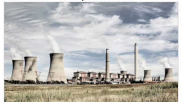
6 Matla STPP Unit 3, Unit 6
