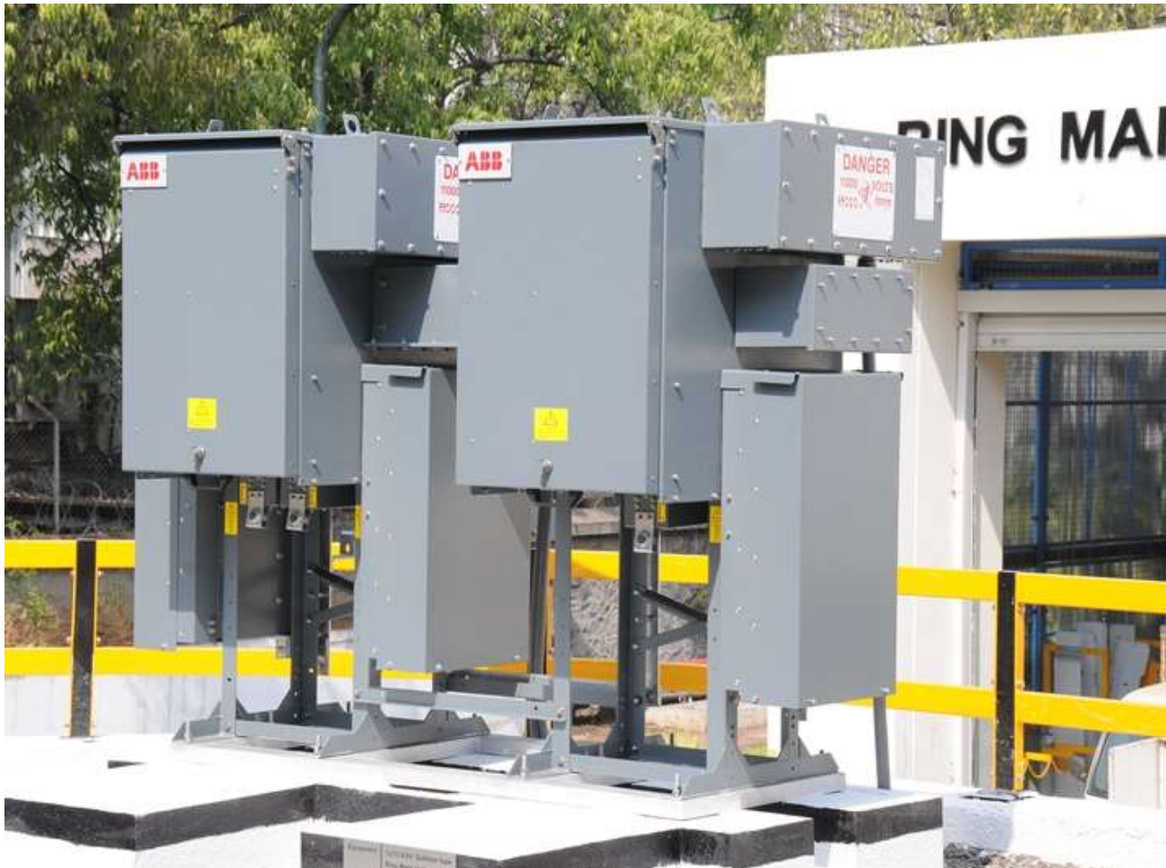
Ring Main Unit – Type- Safe Link- 12kV
