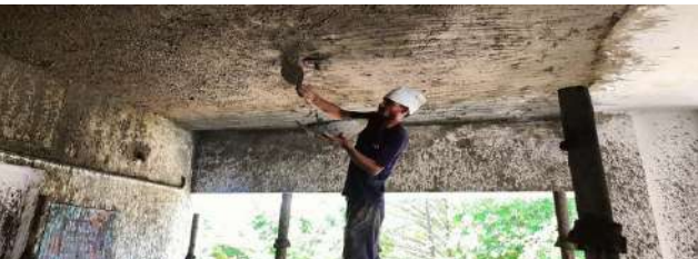
SECOND AND FINAL COAT OF PLASTER
