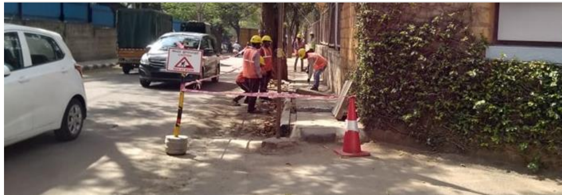
Road infrastructure and public road amenities upgradation in Peenya Industrial area
