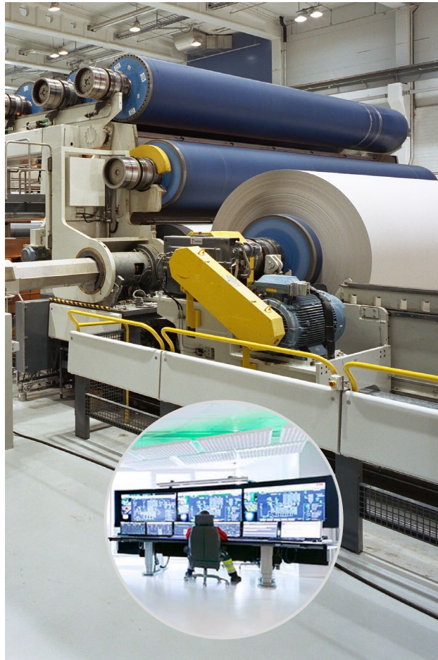
Advanced process control for production at Andhra Paper
