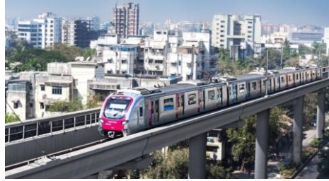
Traction orders including for motors in the metro rail segment in 3 cities
