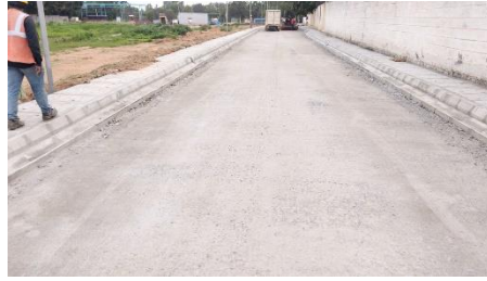
Phase-2 Nelamangala rural road upgradation project - nearing completion
