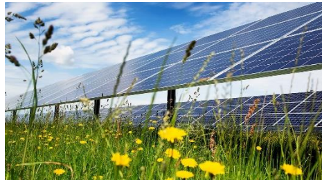
AIS for a 4GW solar project in one of the largest solar parks in Gujarat
