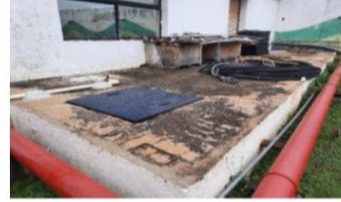
3R - Rain water usage
