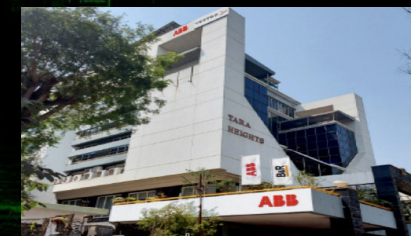
B&R Industrial Automation, Pune*
