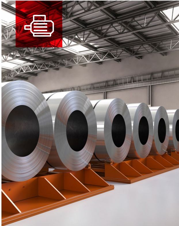
Intelligent motor control center for metal major
