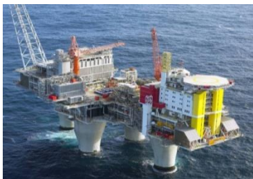
Troll 1 & 3 80+80 MW HVDC Power from shore
