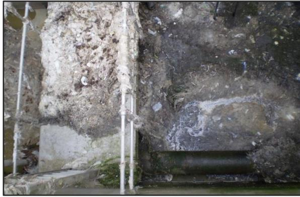
**Caption:** Anglian Water was suffering frequent ragging of its dry well pumps – ragging is where rags foul the pump inlet and prevent the pump from operating normally.
