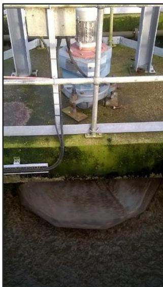
**Caption:** Anglian Water has halved aerator energy costs at the Swallow unmanned treatment works in Lincolnshire by installing an ABB variable speed drive.
