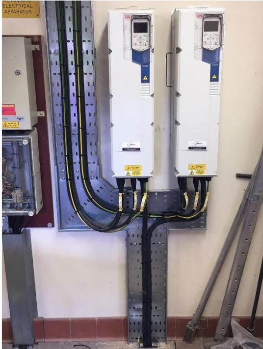
**Caption:** Replacing four fixed-speed pumps with two variable speed-controlled pumps has reduced Anglian Water's annual energy costs by an estimated £4,000
