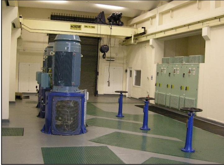
**Caption:** ABB drives help Bristol Water improve the energy efficiency of its pumping equipment at its Purton pumping station.
