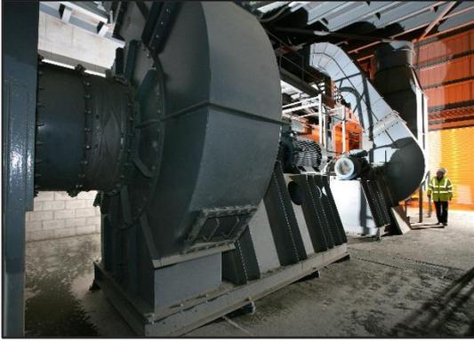
**Caption:** A 2MW ABB industrial drive controls the speed of a large fan that draws air through the 65 metre long kiln.
