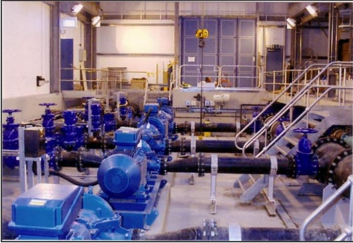
**Caption:** Variable speed drives from ABB are helping to prevent water hammer at Howden Water Treatment Works in Scotland.
