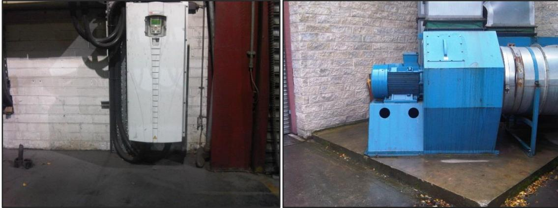
**Caption:** A specialist metal forging company is saving 20 percent on the energy use for its dust extraction system after installing an ABB variable speed drive.
