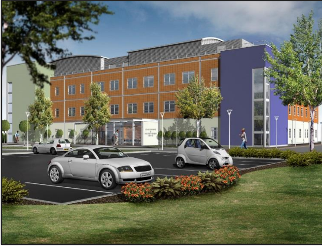
Caption: Ease of integration with building management systems has led to ABB HVAC drives being installed at the new Cheshire and Merseyside NHS Treatment Centre based at Halton Hospital.
