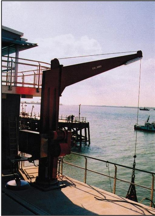
**Caption:** The quayside cranes used by the RNLI, known as davits, have traditionally been manually operated but will now be powered by drives and motors from ABB.
