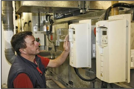
**Caption:** ABB drives control the fans for the air conditioning system serving the two buildings that comprise the stadium's Quadrant expansion project.
