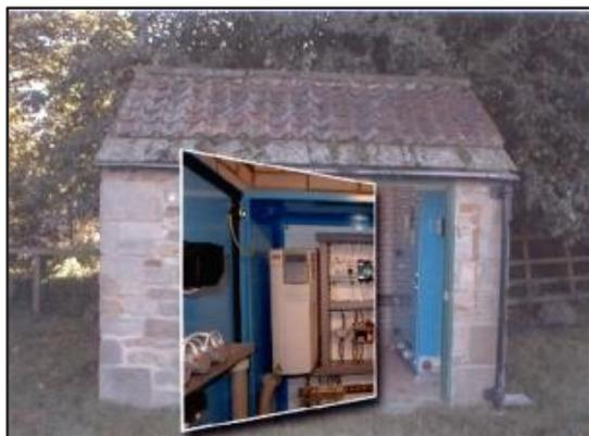
**Caption:** An ABB drive, supplied by ABB Drives Alliance member Slater Drive Systems, is helping Northumbrian Water to save up to £50,000 by running its 3-phase equipment from a 2-phase supply.
