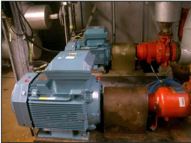
**Caption:** ABB motor and variable speed drives are saving Pfizer €28,000 a year on electricity costs for its chiller applications at its Ringaskiddy plant.
