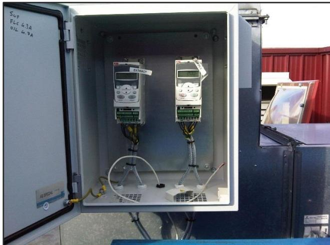
**Caption:** The ABB component drives, installed by Food Industry Technical (FIT), control air supply and extraction by monitoring carbon dioxide (CO<sub>2</sub>) and temperature in the kitchen.
