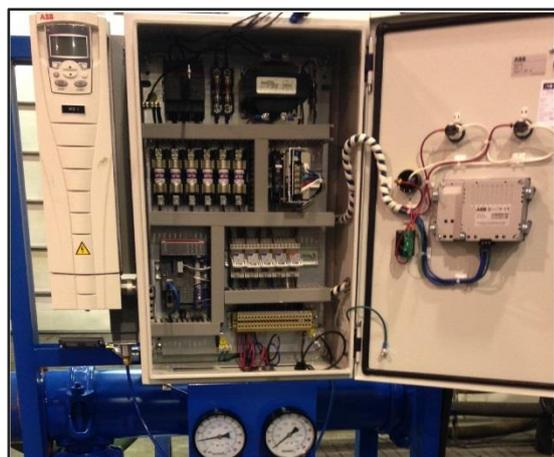
**Caption:** The configuration flexibility built into the control system software that ABB provides makes it easy for Plad Equipment to optimise the pumping systems for each individual action, with variable speed drive, PLC, HMI, Pilot device and protection circuit.
