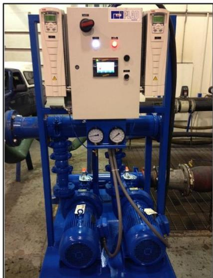
**Caption:** A typical skid mounted booster pump installation from Plad Equipment, with dual pumps and a custom made control panel based on a combination of ABB drives and PLC.
