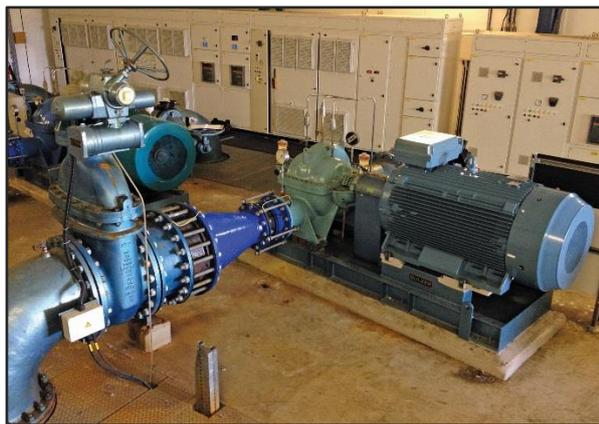
**Caption:** Scottish Water has cut the risk of pump set failure at its Mannofield water treatment works with the installation of an ABB motor and low harmonic variable speed drive.
