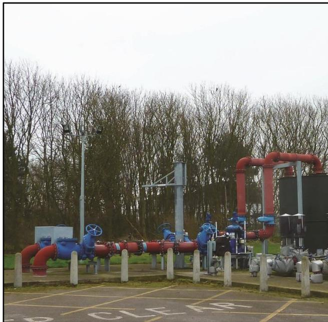
**Caption:** Severn Trent Water has cut the risk of flooding homes with sewerage overflow by installing an ABB variable speed drive within a pump control system.
