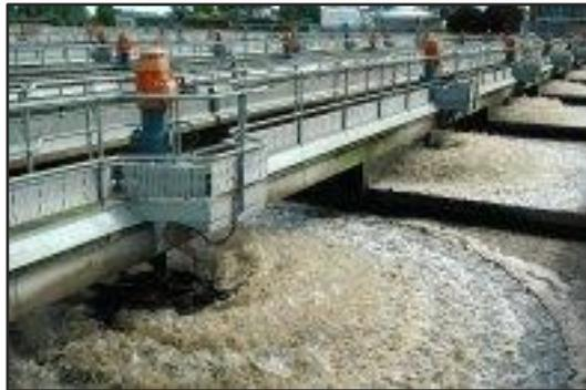
**Caption:** Severn Trent has set up an Energy Saving Project Group to look at replacing and upgrading existing drives, following the replacement of three, 37kW AC drives on water process pumps which gave energy savings of over 65% and a payback of only seven months.
