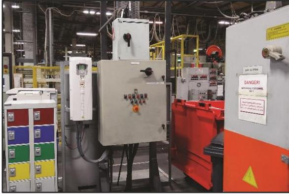
**Caption:** Smurfit Kappa is set to save £60,000 on energy costs following the installation of ABB variable speed drives on its shredder fans.
