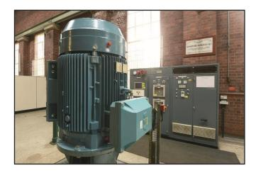
Caption: The world's first IE4 synchronous reluctance motor and drive package from ABB is saving South Staffs Water an additional 6 percent.
