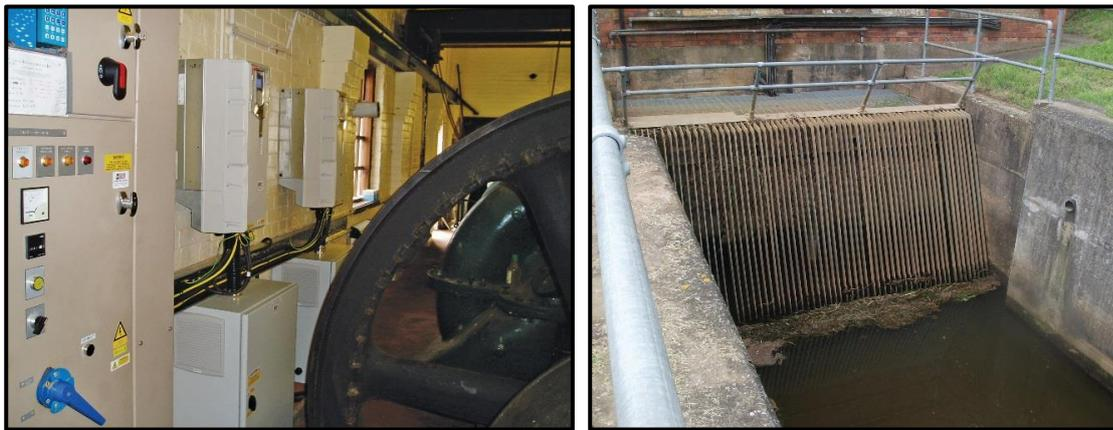
**Caption:** Susworth Pumping Station expects to cut the energy use of two submersible pumps by between 10 and 15 percent following the installation of ABB variable speed drives.
