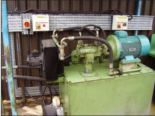
**Caption:** An ABB variable speed drive, designed into a hydraulic system , is saving Trelleborg Sealing Solutions over £12,000 a year on energy costs.
