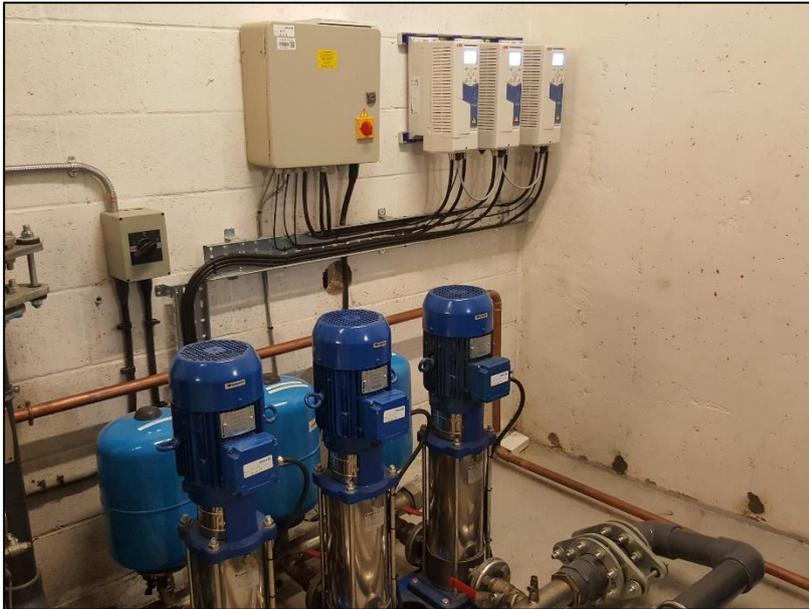
**Caption:** Replacing inverters integrated into OEM-built pump booster sets with variable speed drives, has saved the building's clientele more than £20,000
