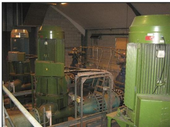
**Caption:** United Utilities’ Drummers Lane water pumping station is saving over £19,000 per year on energy costs following the replacement of its Heenan variable speed drives with new drives from ABB.
